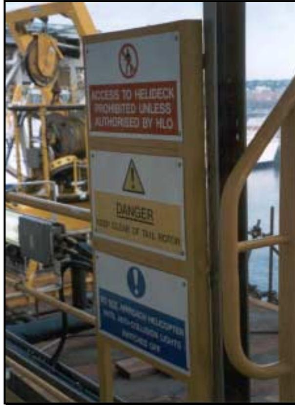
**Figure 7.24 Example of Helideck Safety Signs Securely Mounted on a Robust Frame**
