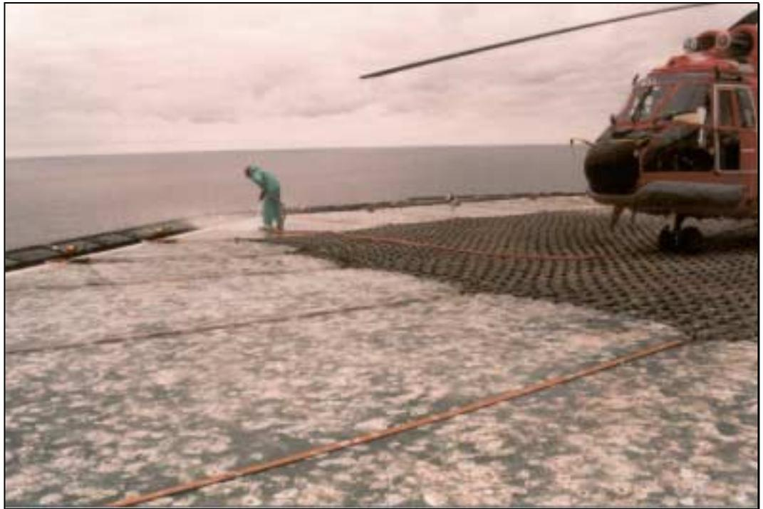
**Figure 10.2 An Example of the Effects of Guano Infestations on a Helideck Surface**
